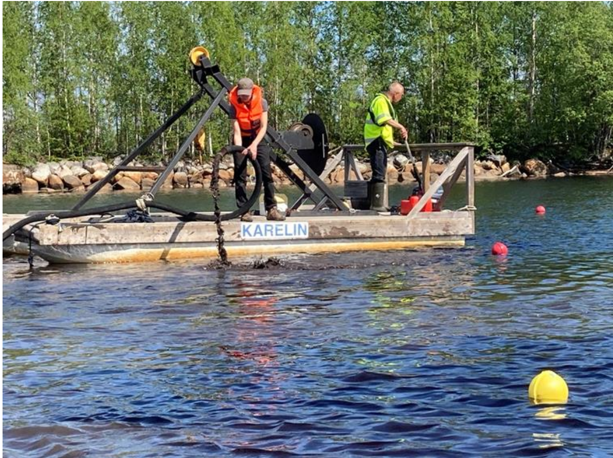
Figure 2 The floating dock was used to monitor the tube that spread the biochar mixture. Anchored floats marked the outer boundaries of the area (Maurice, 2021)
