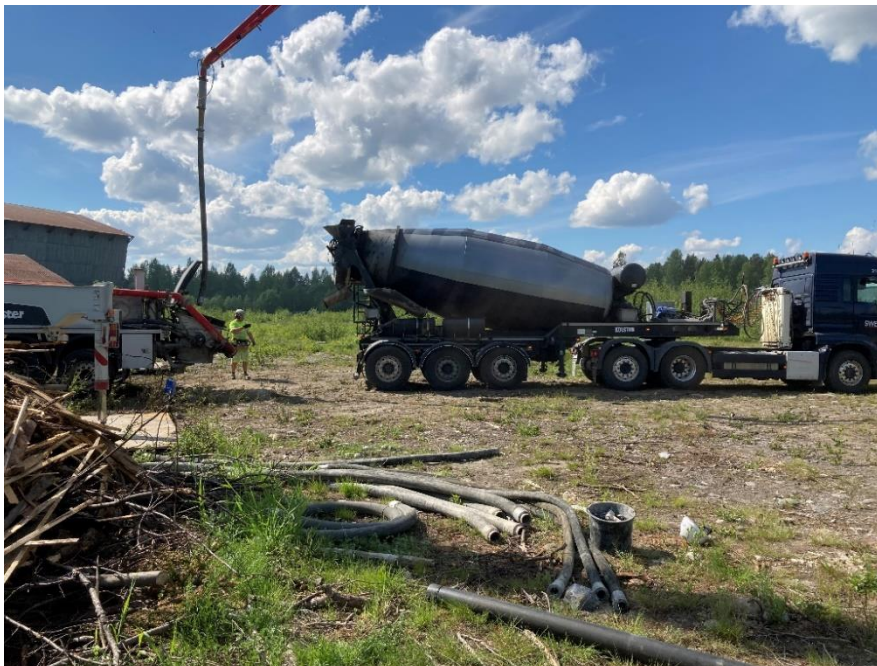
Figure 8. The cement truck that arrived to Bureå with the biochar-mixture (Flodin, 2021).
